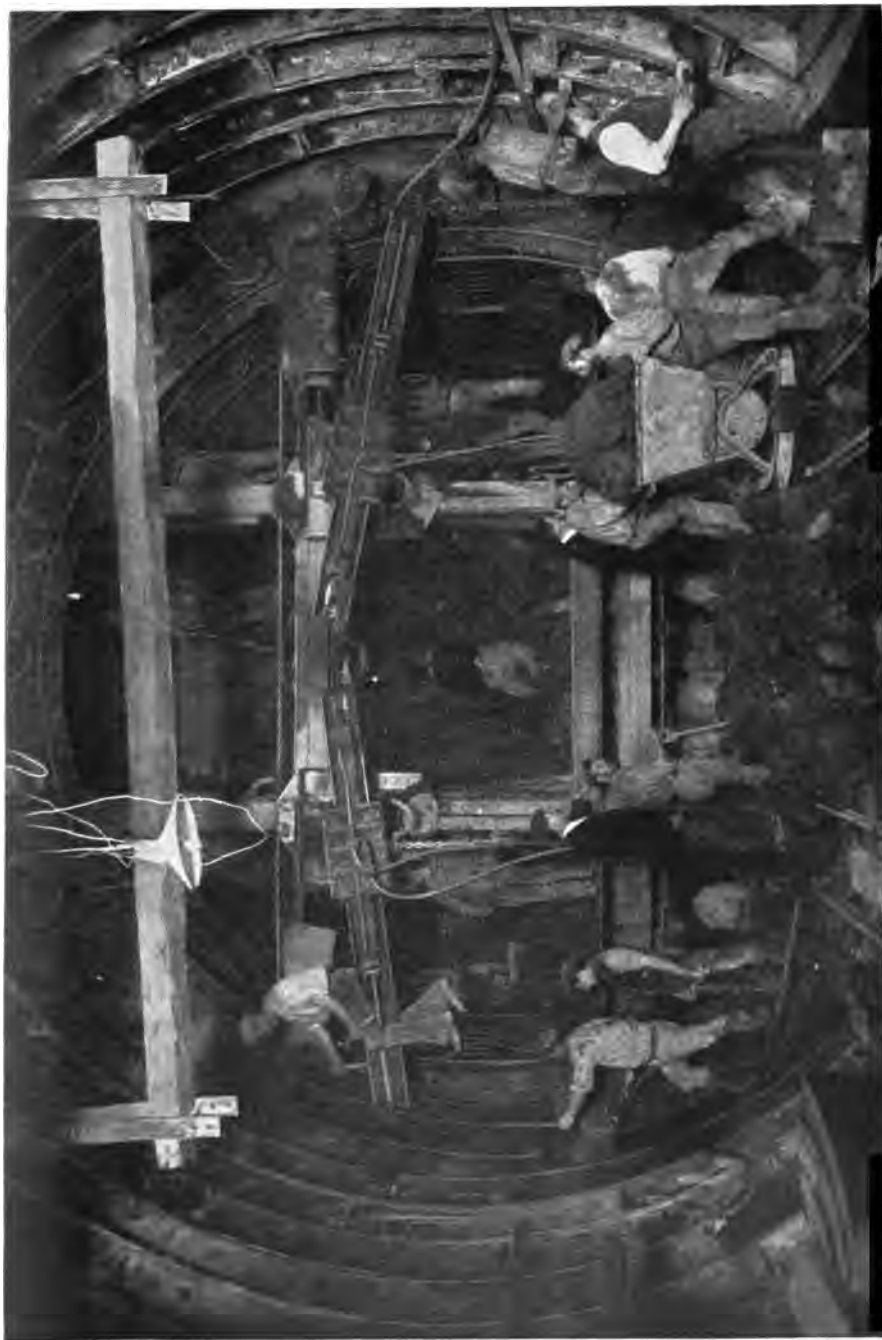
FIG. 13. SHIELD AT WORK IN A TUBE RUNNING TUNNEL
